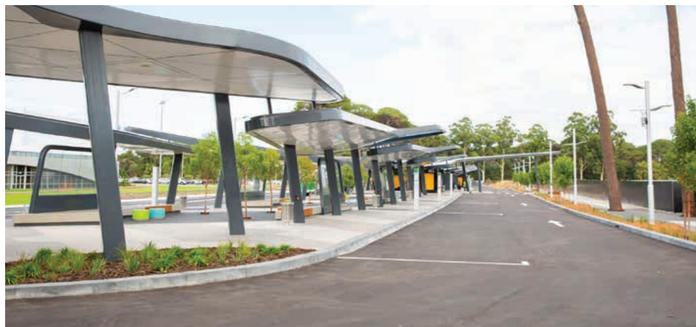
The new Curtin Bus Interchange will commence operation early in 2019.
